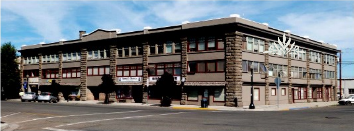
Mercantile and Milling Company Building, Enterprise
