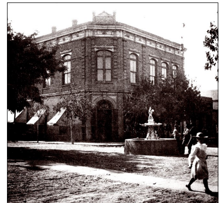
Farmer’s Bank of Weston. Note the architectural cast iron prominent on the building. Fountain in the center of the intersection of Main Street. Photo Weston Public Library 100-05 Bank and Fountain.
