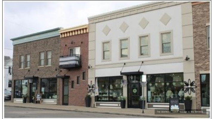
The Daisy in Cedar Rapids, Iowa, operates on the ground-floor of a mixed-use building with upper-story housing.
