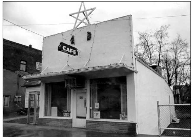
1982: D and F Cafe (Inventory #12), Main Street facade and west side elevation. This building, dating from ca. 1912, is a wood frame structure with "boom town" front which was stuccoed and modified with canopy, plate glass and brick-veneered bulkheads ca. 1956. To left, set back from Main Street, the frame cottage housing the City Library is visible.
