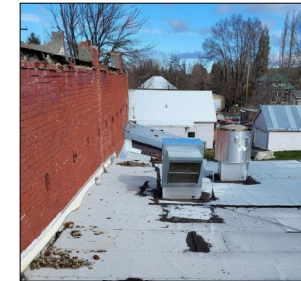
East Wall and Roof over
