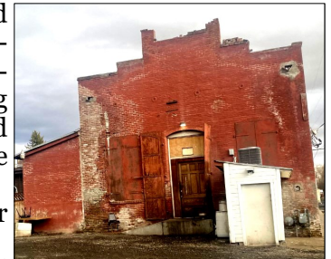
North Wall—note iron shutters at the back door.
