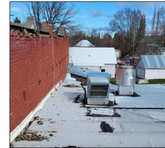
East Wall and Roof over bar.
