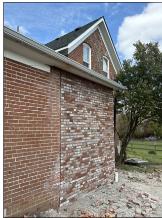
Completed repair of section of house.
