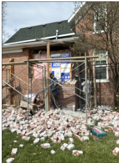
Rebuilding the brick wall.
