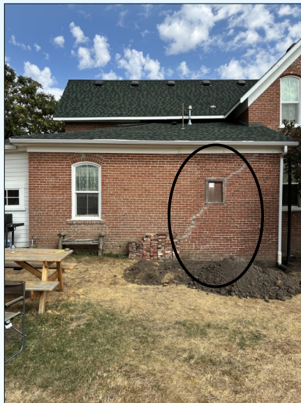
Photo of crack in brick wall of the addition.
