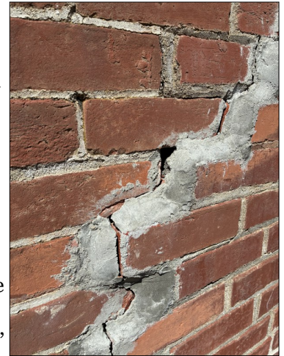
Close up of brick wall.
