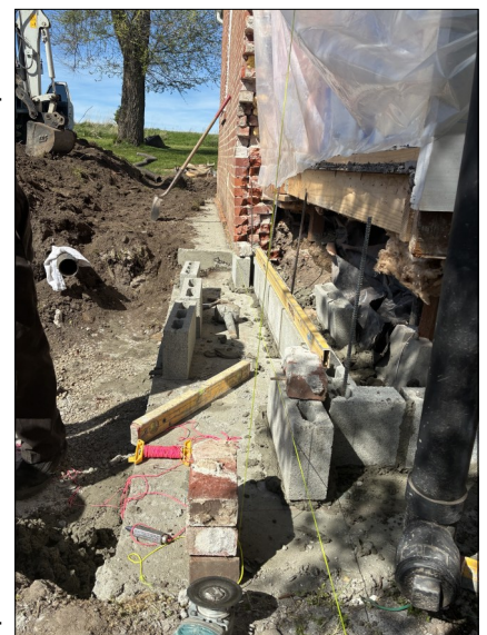
Detailed view of rebuilding the brick wall.
