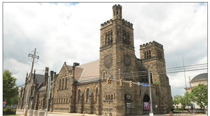
The north and east elevations of New Life at Calvary (Cleveland, Ohio). Two of the roofs in poor condition were discovered at the top of the towers. photo by:Kreative Kage Photographer
