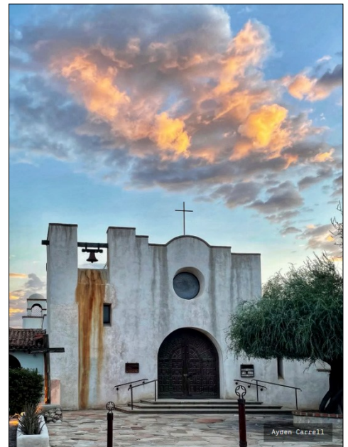
The south wall of Saint Philip's in the Hills Episcopal Church (Tucson, Arizona) where the structural engineer designed a steel channel to be installed along the top of the wall to reconnect the adobe to the roof structure. photo by: Ayden Carrell
