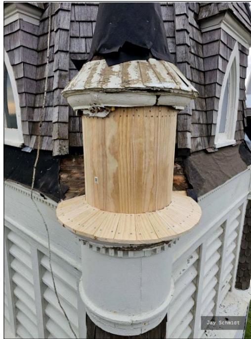
The reconstructed wood turret on the steeple at Vang Lutheran Church (Dennison, Minnesota). photo by: Jay Schmidt
